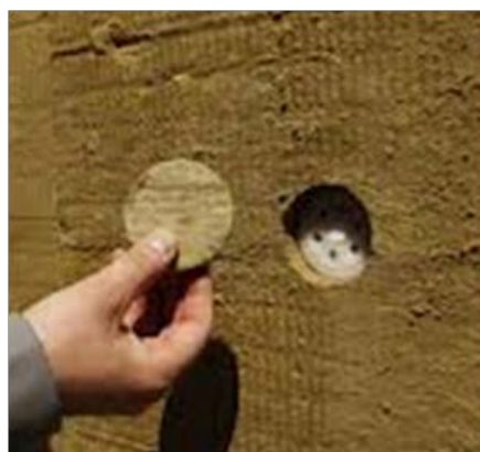
Plugging the anchor with wool
