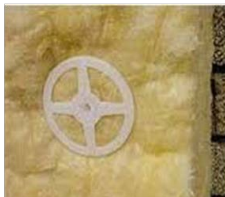
Anchored wool thermal insulation
