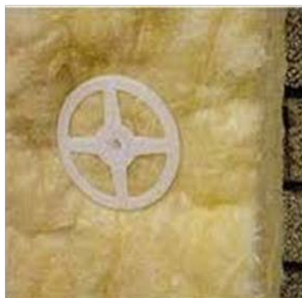
Anchored wool thermal insulation
