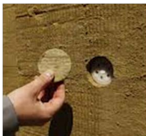
Plugging the anchor with wool
