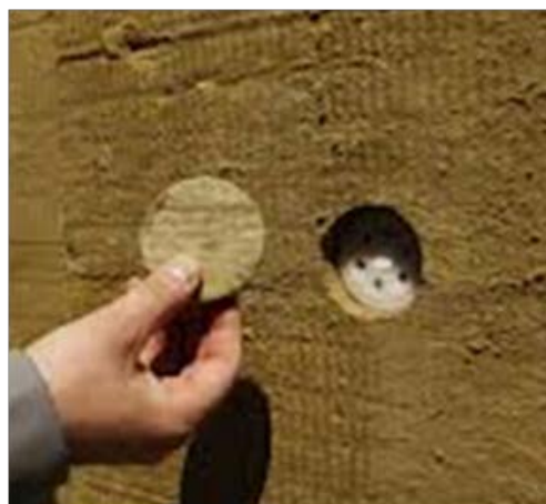
Plugging the anchor with wool
