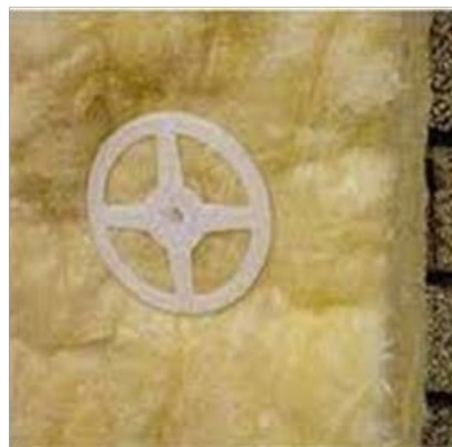
Anchored wool thermal insulation
