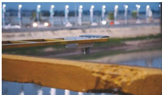
**Photo 3:** An automated water gauge, installed by PIN in Kampong Thom, measures river height with sensor technology. **Photo credit:** Blake Gardiner, PIN
